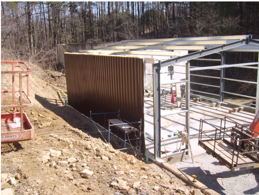
New Steel Building Under Construction on the Upper Drying Bed
