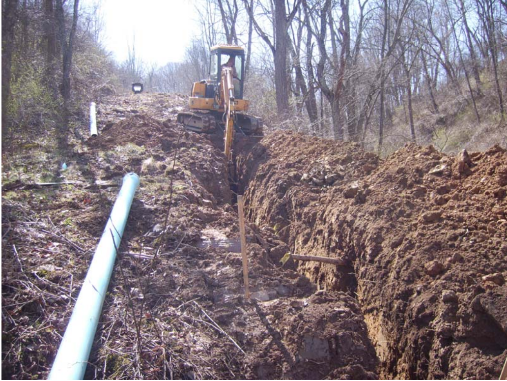
WTP Wastewater Force Main Installation
