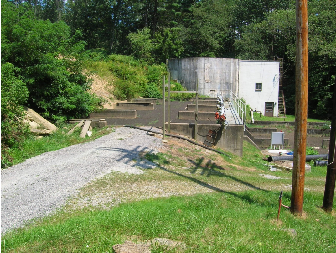
Old Sludge Drying Beds
