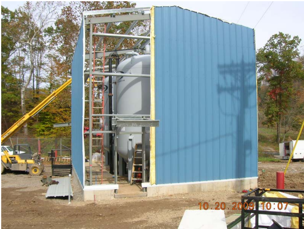
Steel Building Constructed Around Filters
